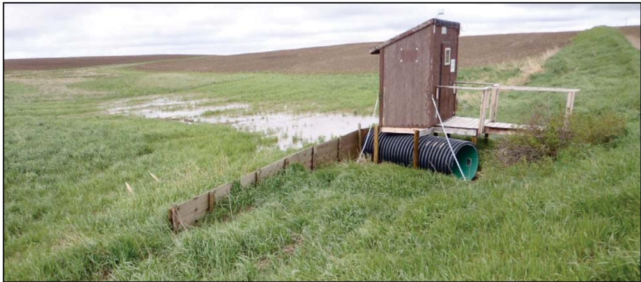
Figure 5.11. Rainfall runoff entering the flume at the edge-of-field monitoring station at the Lower Little Bow River Field site on May 28, 2010.
