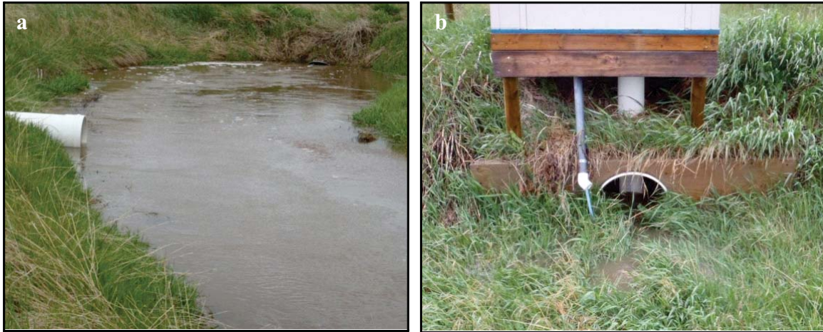
Figure 4.11. Station 204 in May 2010 showing (a) water from the Battersea Drain entering the outlet of the flume and (b) the flume inlet with standing water from the drain.
