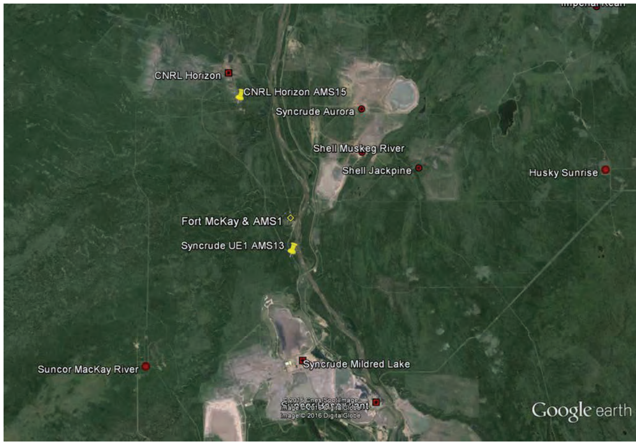
Figure 2: The Location of the CNRL Horizon Air Monitoring Station (which triggered the orange management level under the CAAQS for the LAR) in Relation to Area Oil Sands Developments, Fort McKay, and the Fort McKay and the Syncrude UE1 Air Monitoring Stations
