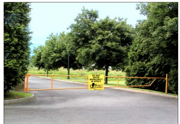
Figure 3 Tapered Metal Pipe Gate
