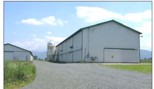
Trees and Shrubs Kept Away from Barn
