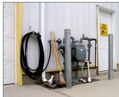
Water Source Readily Available
