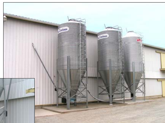
Clean Feed Storage Area
