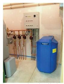
In a recent study conducted by the Canadian BioEnergy Centre (CBEC) at UNB, a 56 kW state-of-the-art pellet-fired hot water heating system was installed at a local rural New Brunswick recreational hall and monitored over a one-year period.
